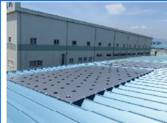
● 施工後 / After installation
